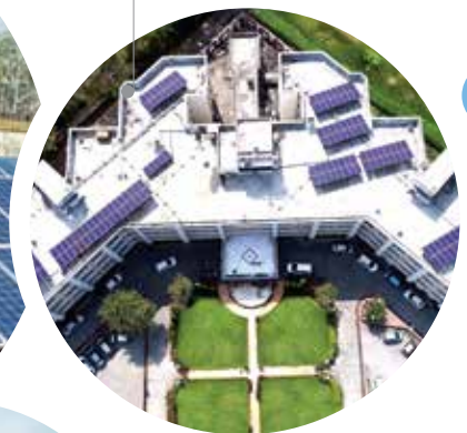
● GST Bhavan, Vadodara 100 kW
